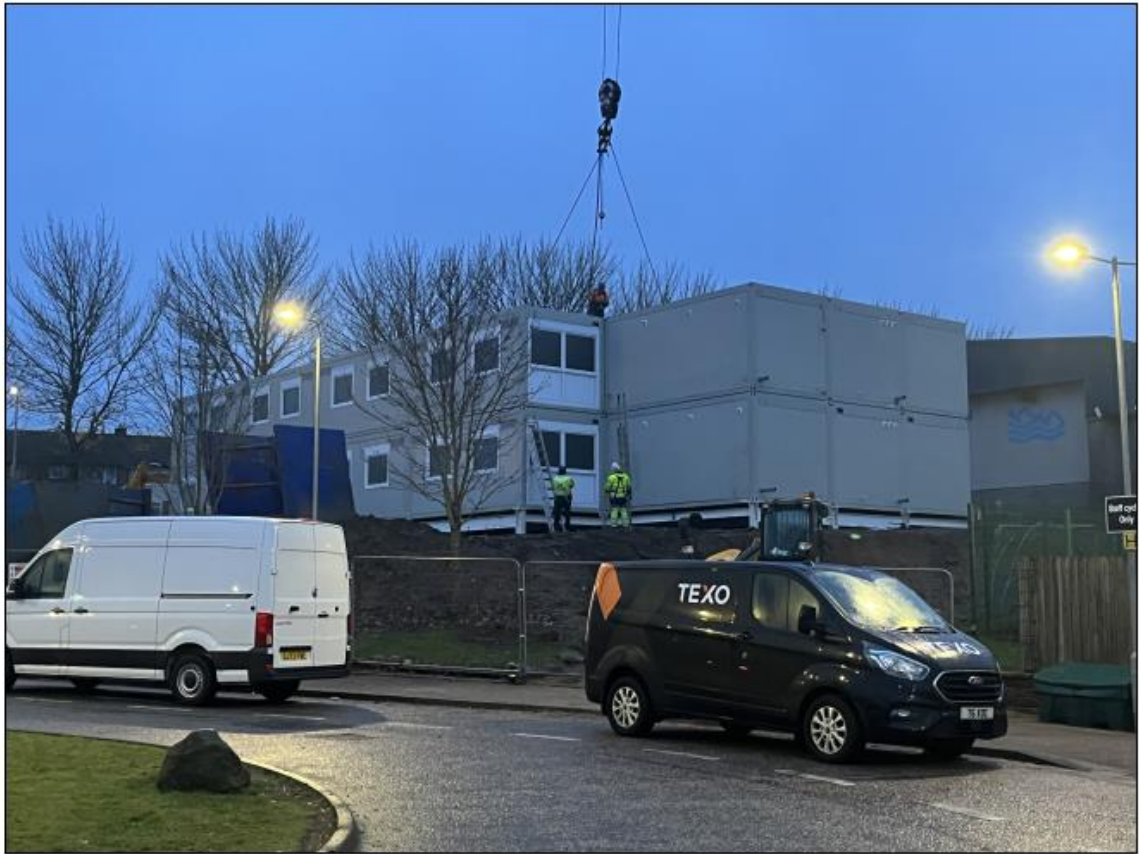
Installation of the units
